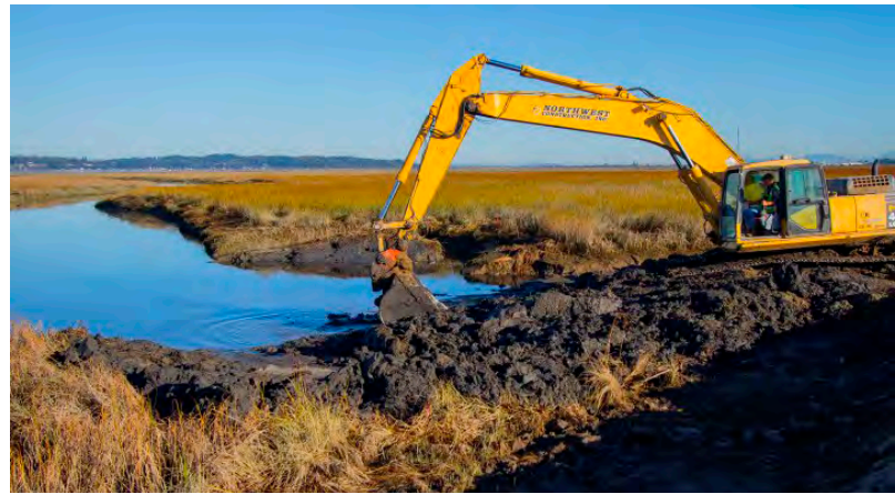
A backhoe works to bring the dike down to marsh level and open a channel for tidewaters to flow into the marsh at Port Susan Bay, Washington. Photo: Nature Conservancy. Copyright: Marlin Greene/OneEarthImages
