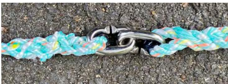
Pretension is needed to reduce growline sag between the set line flotation. Deadeye tensioners were added to each of the ten anchor lines to allow each to be adjusted as needed.
